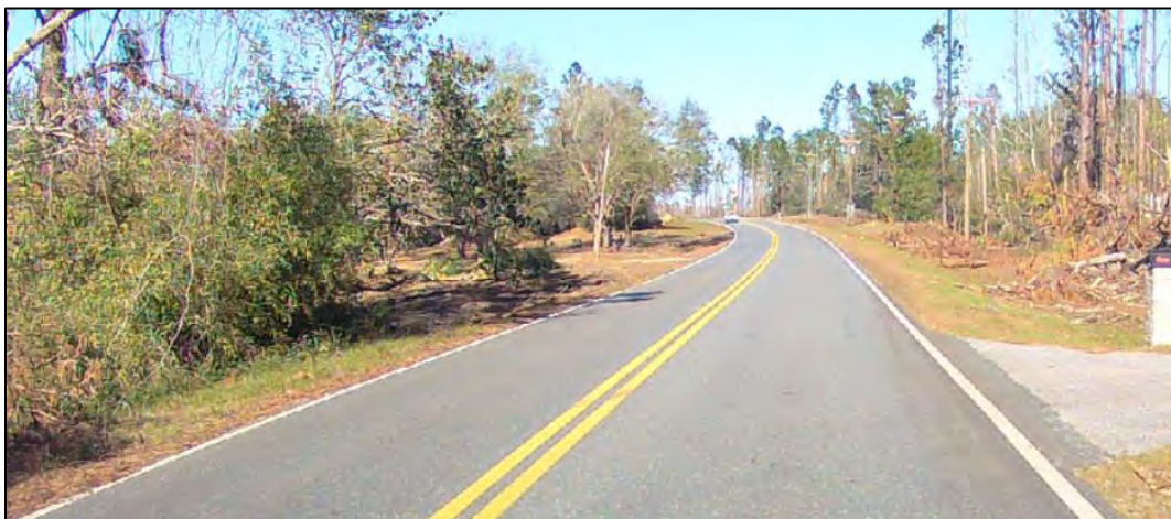
Figure 34. Restricted sight distance between vehicles approaching from S and E
