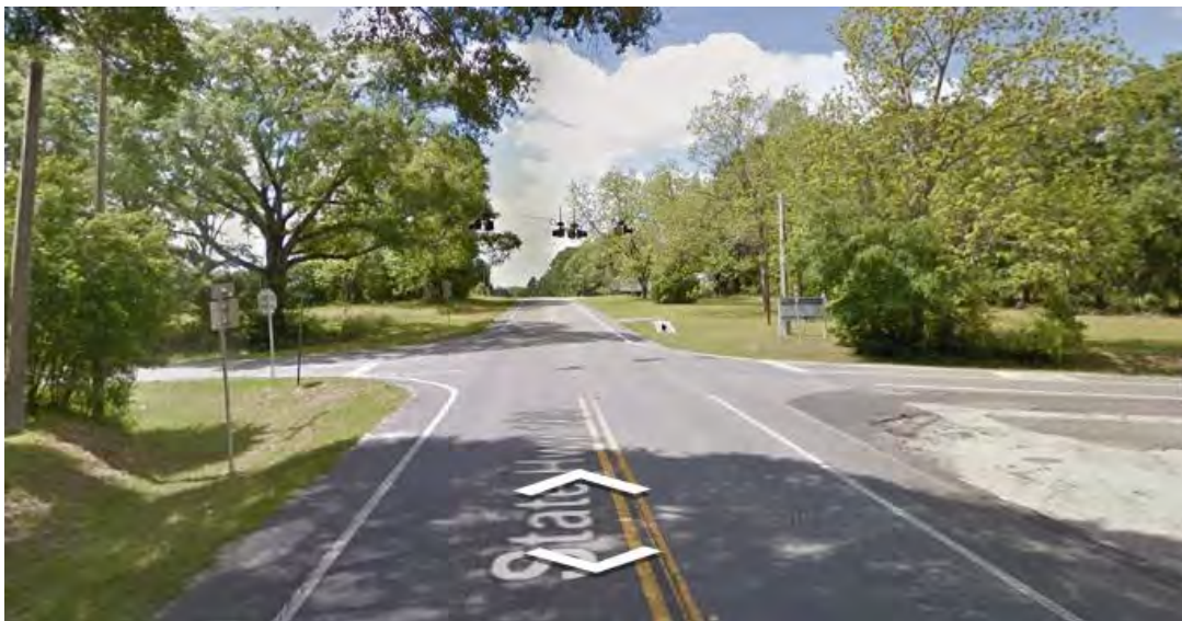
Figure 24. Visual obstruction due to hill at intersection of CR-164 and SR-273
