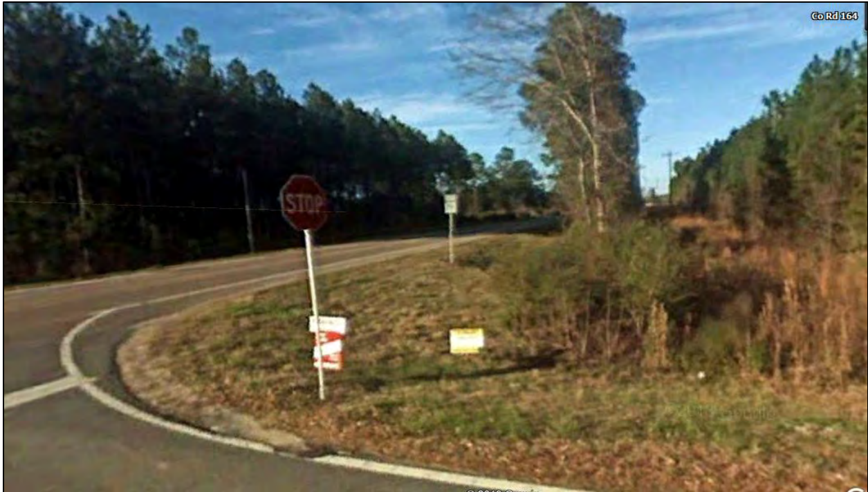
Figure 23. Visual obstruction at intersection of CR-164 and SR-77
