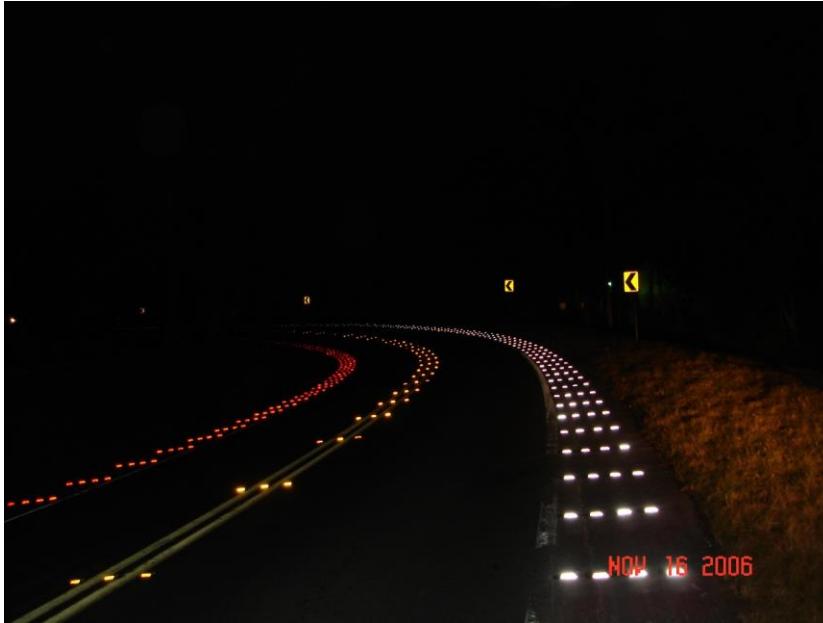
Figure 9 Enhancement of nighttime visibility of a curve using raised pavement markers on shoulders
