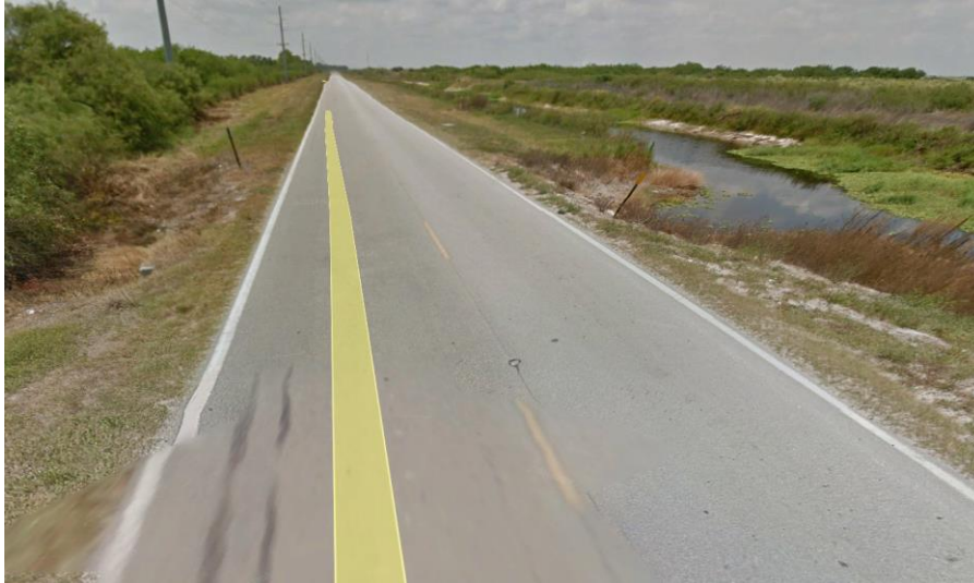
Figure 27 Canal crossing without guardrail on CR 835
