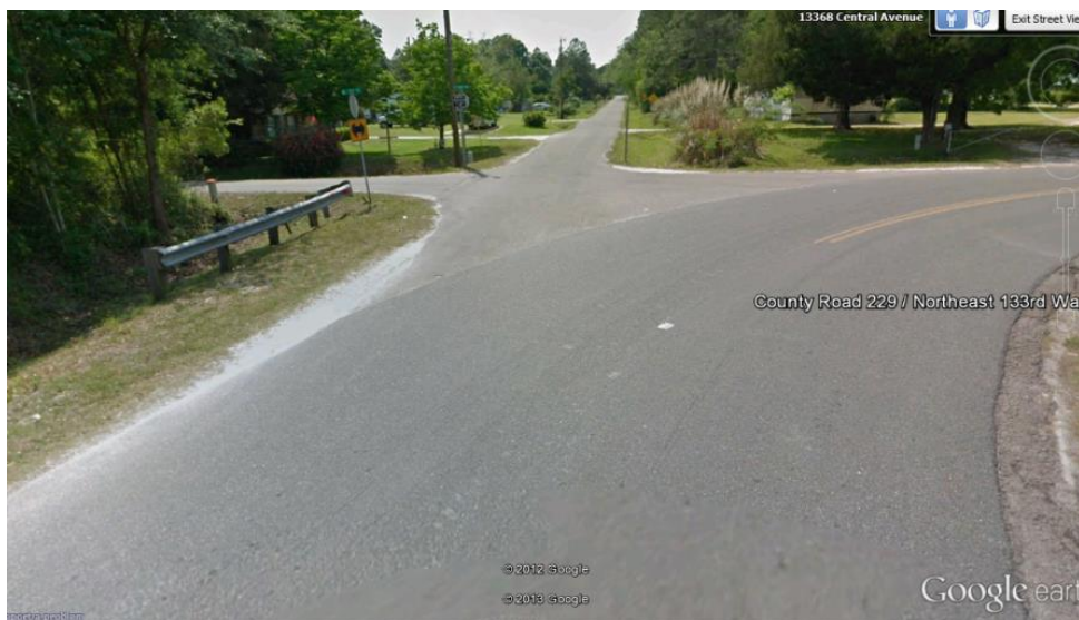
Figure 17. Westbound view showing lack of signage delineating turn at NE 228th Place/NE 125th Way
